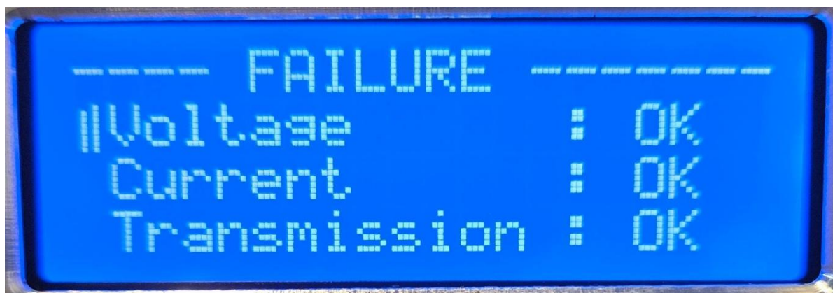
Figure 82. Front panel display – failure Current
