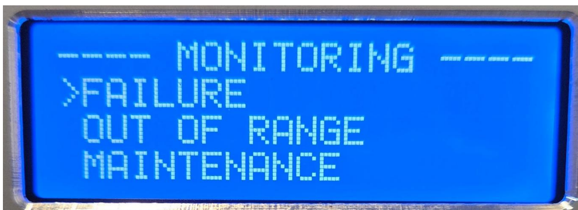
Figure 77. Front panel display – monitoring.
